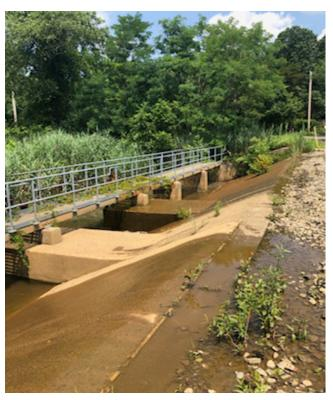
2. Tennent Brook 5 (TB5) is an undersized set of double culverts just downstream of the dam. These culverts were completely submerged during the field assessment, in low-flow conditions, so roadway flooding here is likely.
