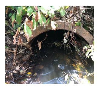
3. Tennent Brook Tributary Bo.5 (TBBo.5) is a severely undersized double culvert that connects Prickets Pond to Tennents Pond. The maximum storm interval that it can accommodate currently is a 1-year storm event, which changes to zero under increased precipitation scenarios indicating certain flooding.
